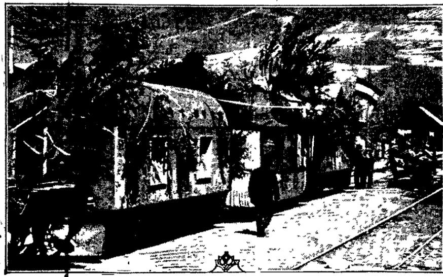
DISGUISED AUSTRIAN ARMORED TRAIN. In the accompanying illustration is shown an armored train of the Austrians bedecked with shrubs and foliage so as to resemble a part of the country through which the train passes. This method of disguise is particularly valuable in protecting the train from aerial attacks. The pilot of a hostile air craft invariably is completely fooled by this ruse.
